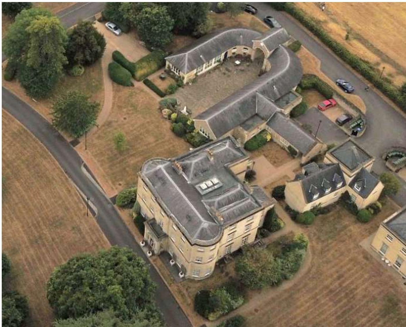
Beechfield House and The Stables
