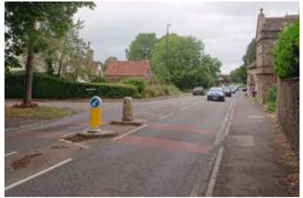
Bollards at Woodlands—the far one not illuminated
