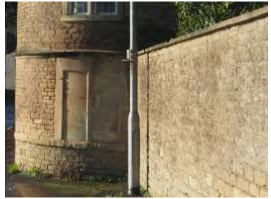
The wall from the Roundhouse to Beechfield
