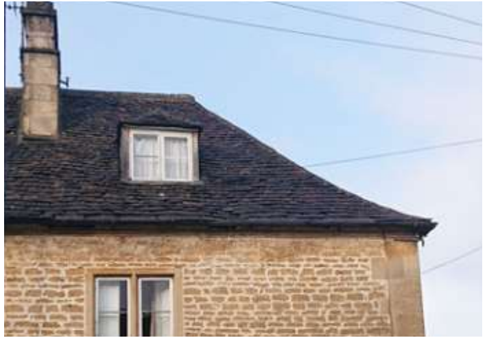
Slight eaves 'bell cast'
