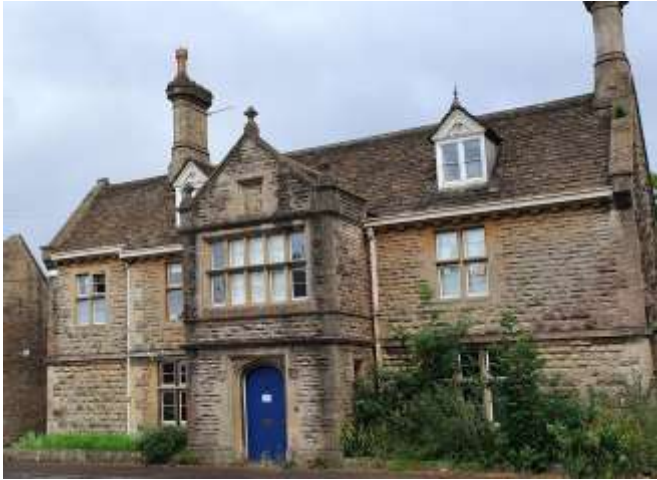
This house is thought to have been built by the Poynders to accommodate their Chaplain who took services at their (still standing) private chapel - Hartham Chapel.
