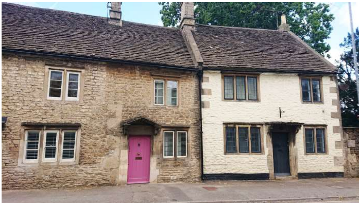
No. 27 squeezed in alongside No. 25
