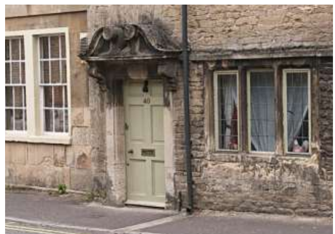
No. 40 Pickwick featuring an elaborate stone hood porch
