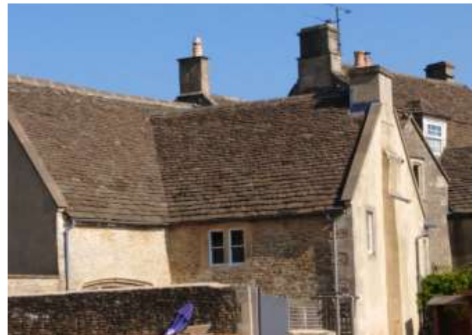
Another rebuilt stump without shaft (on gable at right)
