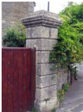
Middlewick Lane gate pillar
